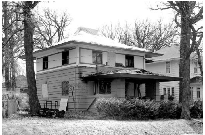
Yelland House, after the fire. Photo courtesy of Bob McCoy
