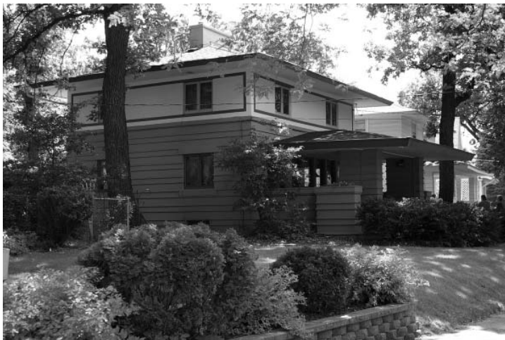
Yelland House, before the fire. Photo courtesy of Bob McCoy
