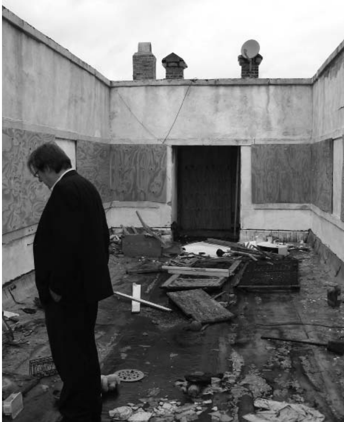
James Weirick on the roof of Griffin's Cornell Store and Flats, 1908. Photo by Paul Kruty.
