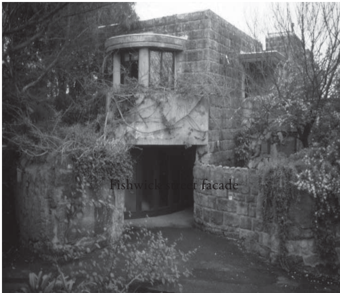
Fishwick street facade
