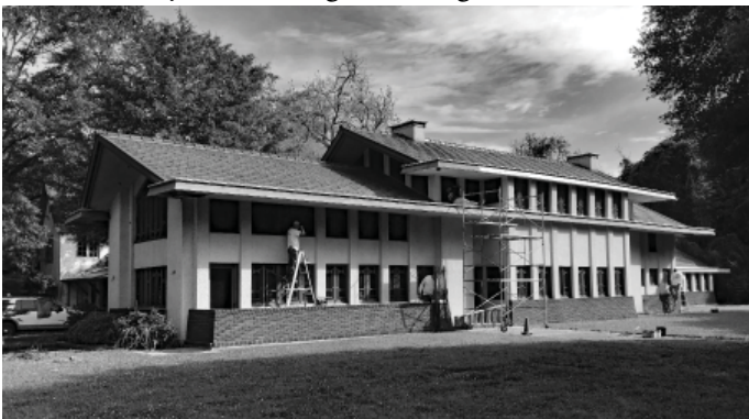
Exterior work on the Cooley house
