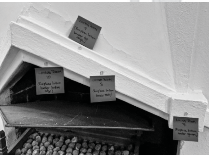
Labeled paint samples at the fireplace
